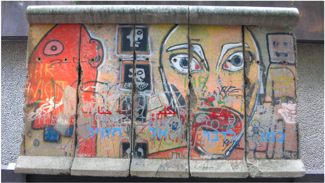
Figure 4 Image of the wall in the courtyard showing the graffiti after the waterfall had been shut off. The area from which the fragment shown in Fig. 3 had detached is seen at the bottom right of the central panel. There are three vertical exposed rebars visible from within the loss. Image: © Tishman Speyer, 2014.
