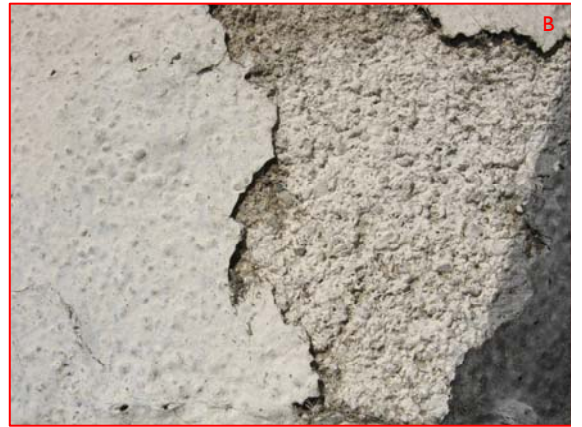
Figure 10.127: Detail; a layer of opaque white paint has been painted over much of the mural's surface to hide existent graffiti marks. Photo: Courtauld Institute CWPD 2007
