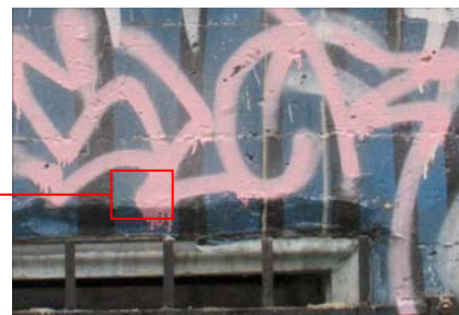
Figure 10.21 (above): Site of trial 102-T.20; pre-cleaning. Photo: Courtauld Institute CWPD 2007
