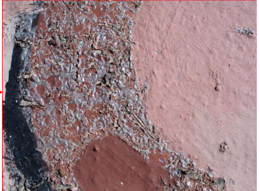
Figures 10.89 (above left) and 10.90 (above right): Detail; north wall. Cracking and flaking of the original paint layer. Photo: Courtauld Institute CWPD 2007
