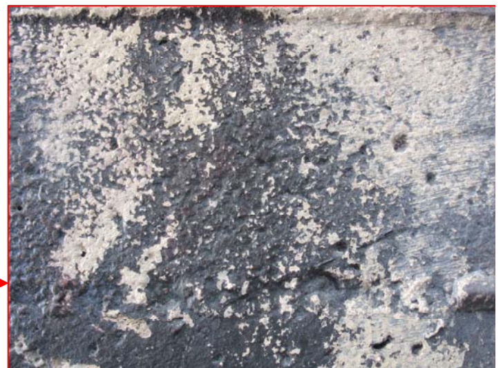
Figures I.21 (above left) and I.22 (above right): Detail of the damage caused to the original paint layer by a poorly implemented attempt at graffiti removal. Photos: Courtauld Institute CWPD 2007.
