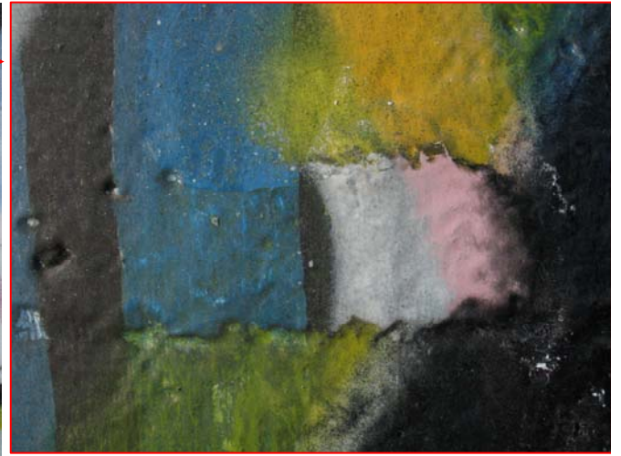
Figure 10.17: Detail; results of cleaning trial 102-T.12 showing excellent removal of the more soluble yellow and black graffiti paint but with no effect on the less soluble white and pink graffiti paints. Photo: Courtauld Institute CWPD 2007
