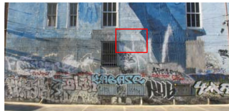
Figure 10.11 (left): The thick gel medium was applied as a coating to the lower half of the mural surface in the late 1970s to protect the surface from graffiti vandalism. Due to its low glass transition temperature the coating has attracted dirt and pollution causing a darkened appearance. Photo: Courtauld Institute CWPD 2007
