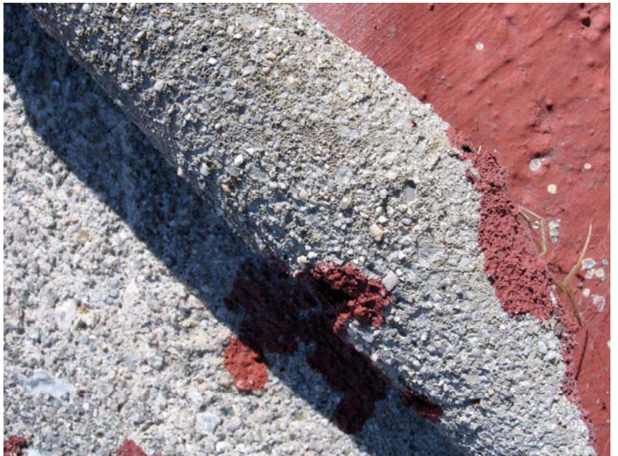
Figures 10.91 (above left) and 10.92 (above right): Detail; north wall. Severe curling of the original paint and preparatory layers. Photo: Courtauld Institute CWPD 2007
