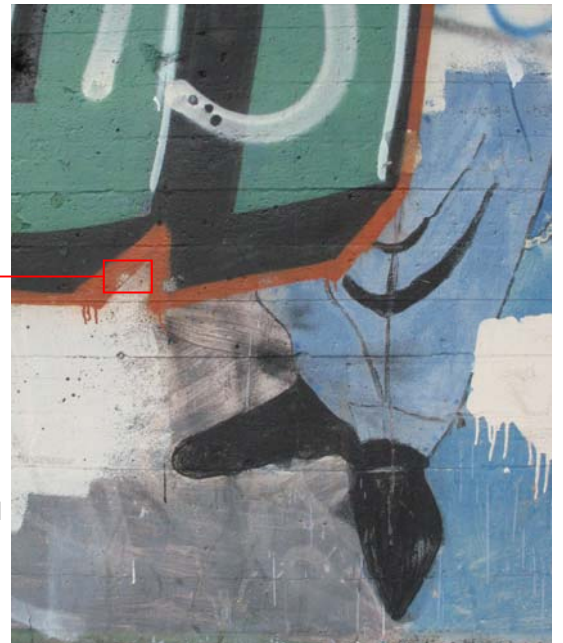
Figure 10.130 (above): Site of the most successful cleaning trial (106-T.04) on the less soluble aerosol graffiti paint. Photo: Courtauld Institute CWPD 2007
